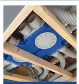
Semi rigid ductwork is ideal for smaller developments.
